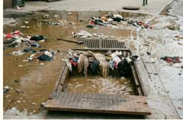
Sewage Pipe Leakage
